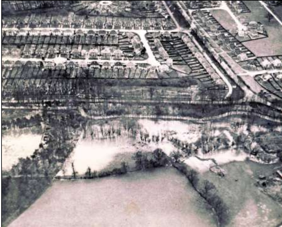
The Hogsmill in Flood 21 July 1937 Worcester Park Road, Kingston Road, Mortimer Crescent
