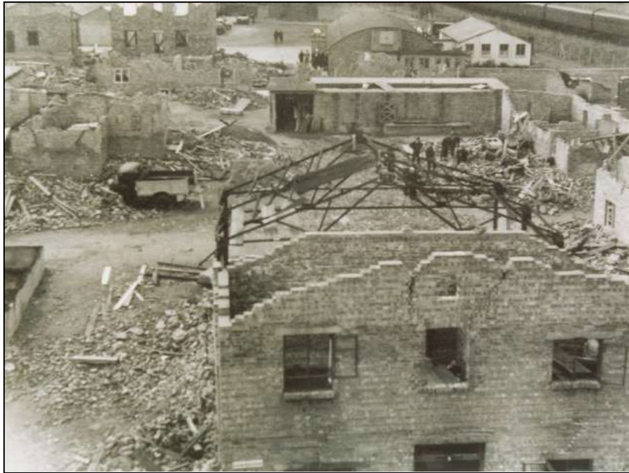
The Civil Defence Training Ground, Kiln Lane, Epsom . Date Not Known
