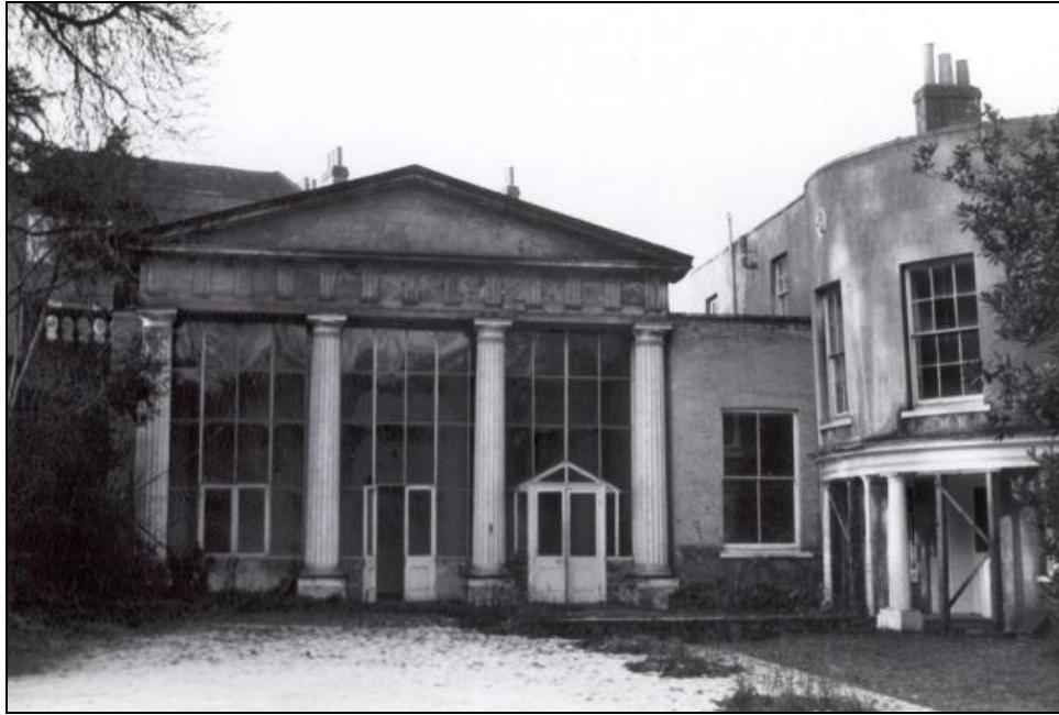
The Doric Columns before demolition. Image courtesy of Bourne Hall Museum.
