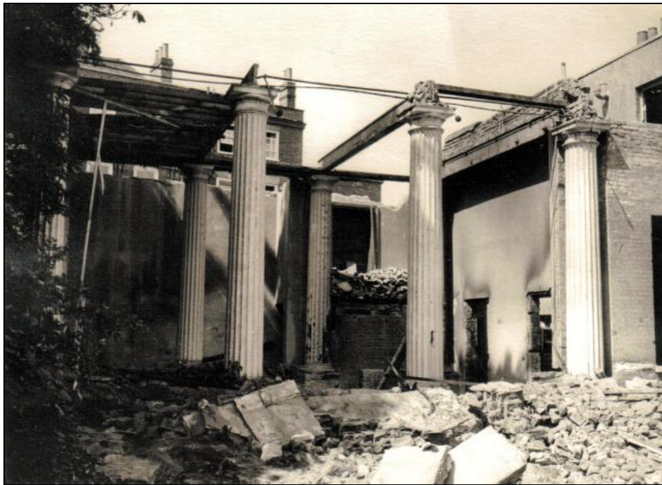
The Doric Columns during demolition photographed in July 1967 by LR James.
