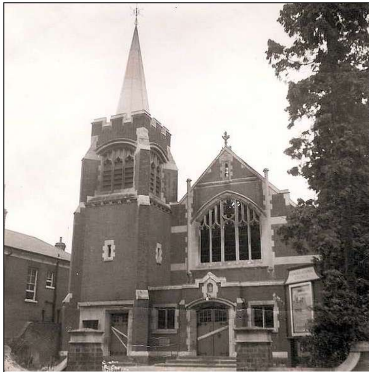
Epsom Congregational Church, Fire Damage West End 1961
