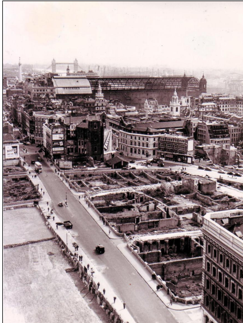
The view from the top of St. Paul's Cathedral (Tower Bridge in the background) overlooking the bomb damage
